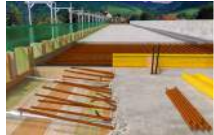
Rebar connections
